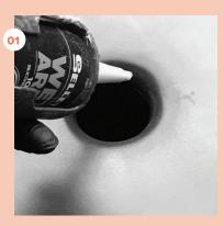
Run a bead of clear wet area silicon around the waste rim
