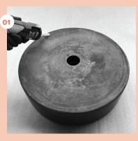
Run a line of clear wet area silicon around the underside of the basin 10mm back from the edge
