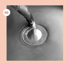
Carefully push silicon around gap between waste and sink
