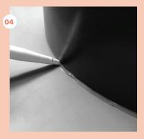
Run a bead of clear wet area silicon to fill the gap between the basin and benchtop
