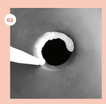
Be generous with application. It is critical that silicon overflows when waste is placed down
