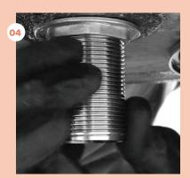
Hand-tighten waste. Do not over tighten.
