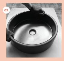
Press down into benchtop and remove excess silicon using wax and grease remover and soft cloth
