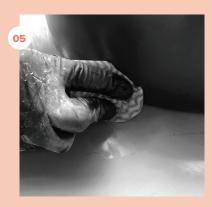
Smooth silicon off to a neat finish and wipe clean with wax and grease remover
